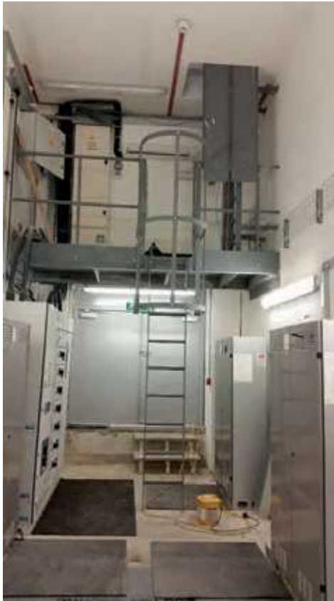
Lower machine room, where a ladder and an intermediate platform reduced the rise to less than 2.5 m to avoid the need to install a stair
